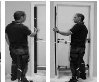
**GB** Secure a wedge to the mitre at the hinge side to fix the frame at the top. Now, make sure the hinge side jamb is perpendicular.
