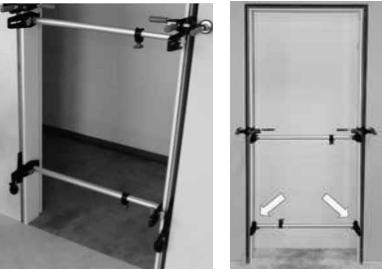
**GB** Place, at the height of the lower mounting spreader, an air cushion between the frame and the wall both left and right, and inflate these so that they cannot drop out.
